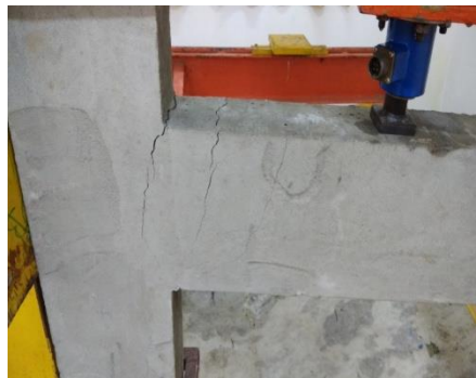
Fig 3.8- Beam-Column Joint –Cracks
