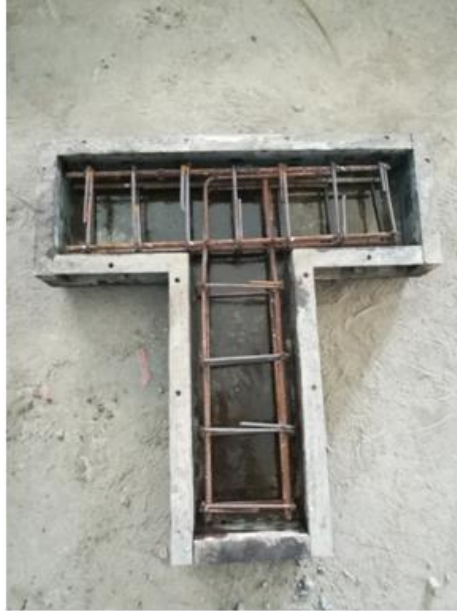
Figure 3.2 –Preparation of mould with reinforcement.
