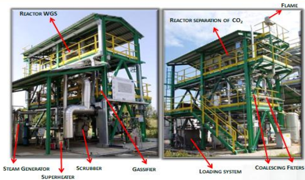
UPDRAFT FIXED BED PLANT OF 150 KWTH
