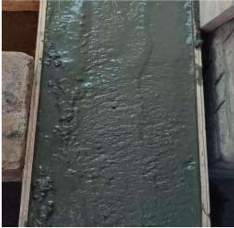
**Fig 3 Retrofitting of beam**
