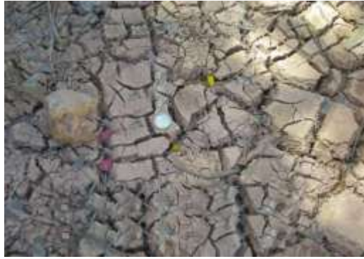
Figure 1: Crack pattern near Kaolin deposit
